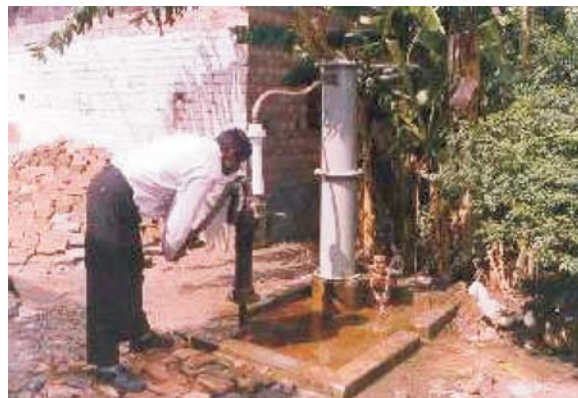
Fig A1.7: Arsenic removal kit with hand pump
