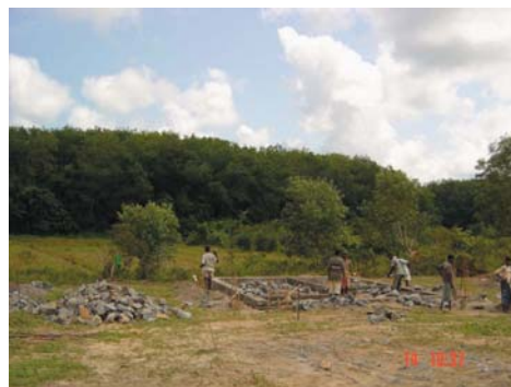
Fig 4.2: The site, before construction began
